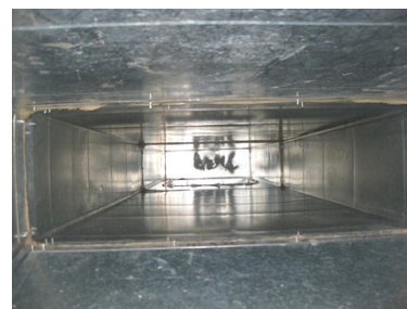
Bright and Shiny Duct work after being cleaned
