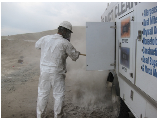
Pictures from the jobsite
